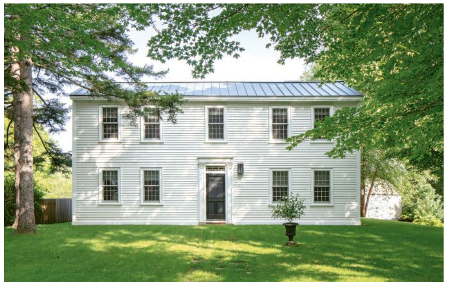
The Federal-style house had been added onto multiple times in its 200-plus years, but only the original portion was salvageable. A revised set of additions follows the path of the old while blazing new trails.
