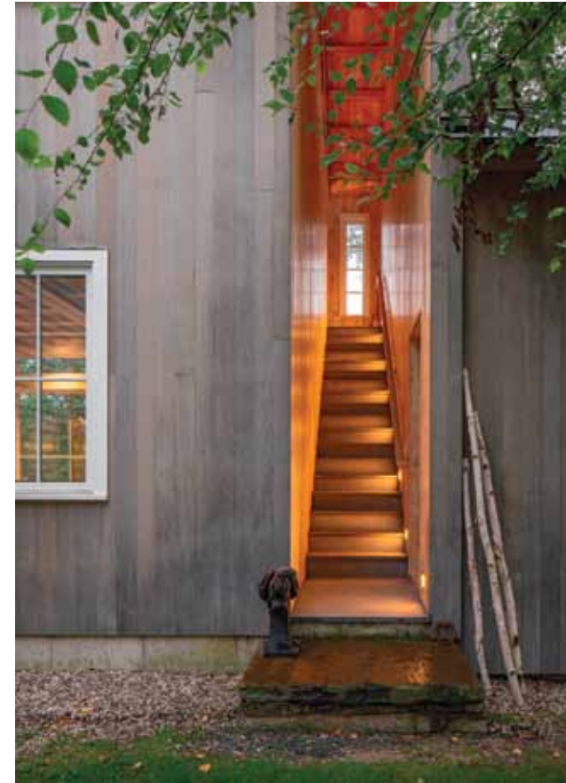
Creating a slot stair. A 38-in.-wide “slot” stair in the studio separates an older restored barn from the new structure. Because Galaxy Schist , a locally sourced stone, was used for the landings, treads, and risers, the stairs needed to be engineered to handle the added weight. The stairwell is clad in whitewashed tongue-and-groove chestnut finished with rubbed urethane.
